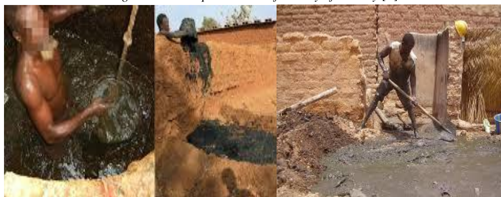
Figure 2: Manual emptying of a latrine
