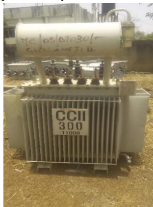
Figure 2: 300 kV transformer showing its conservator tank
